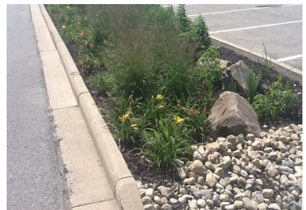
Figure 2: New bioswale installation
